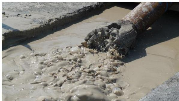
Bentonite drilling fluid
